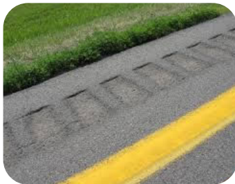
Mumble strips reduce cross centerline crashes.
